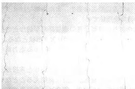
Fig.4 The situation of heat crack
